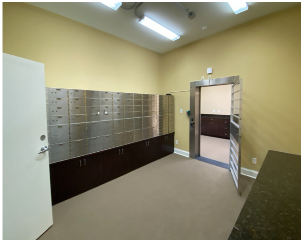
VAULT AND SAFE DEPOSIT BOXES
