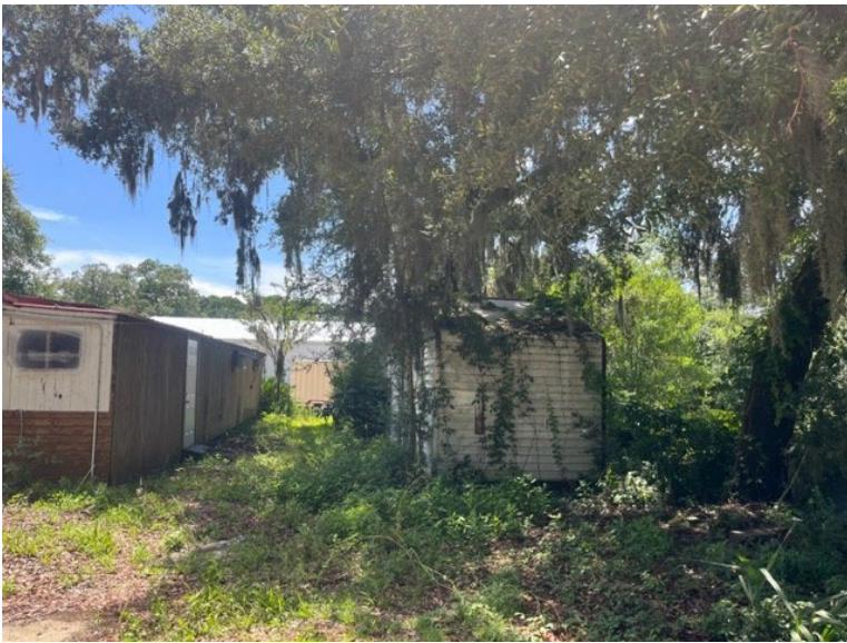
Figure 7 - Existing Accessory Structure
