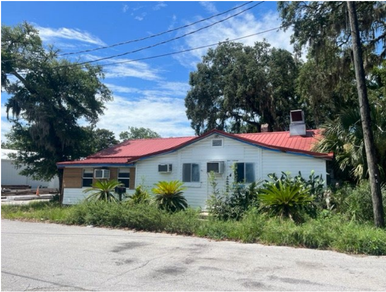
Figure 5 - Existing Structure Frontage
