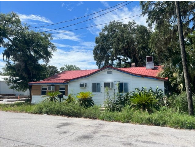
Figure 5 - Existing Structure Frontage
