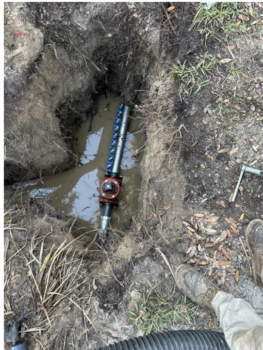
Windy Lane Valve Replacement
