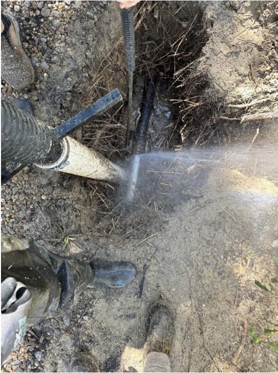
Windy Lane Valve Failure
